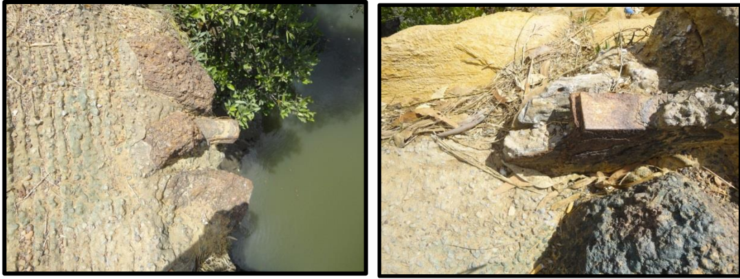
Figure 7.61 Steel beams protruding from asphalt (left and right respectively)
