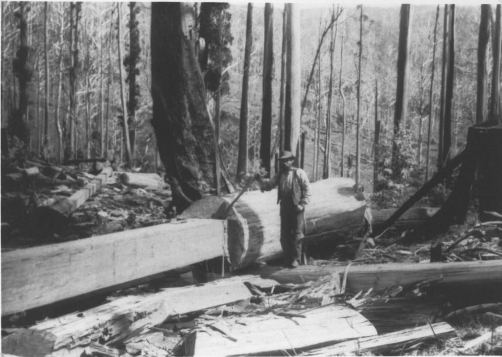
Plate 1 Preparation of a blue gum pile with an adze and broad axe in the 1920s.
