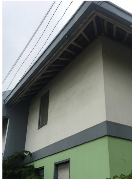
Figure 7. 7: Bamboo providing support for the roof of Dutch Hospitality houses
