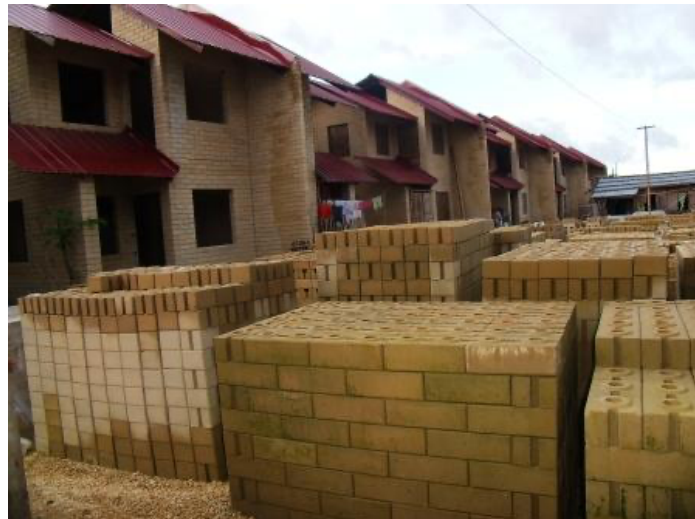
Figure 7. 6: The Interlocking Compressed Earth Blocks used for the construction of Dutch Hospitality houses
